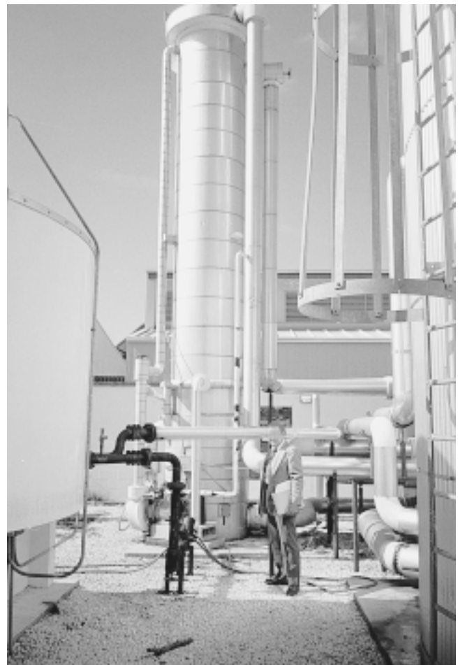
Fig. 17 Separated ice slurry system equipment The tall tower in the center is the evaporator. The ice storage tank is on the right. The chiller condensing unit is on the left.
