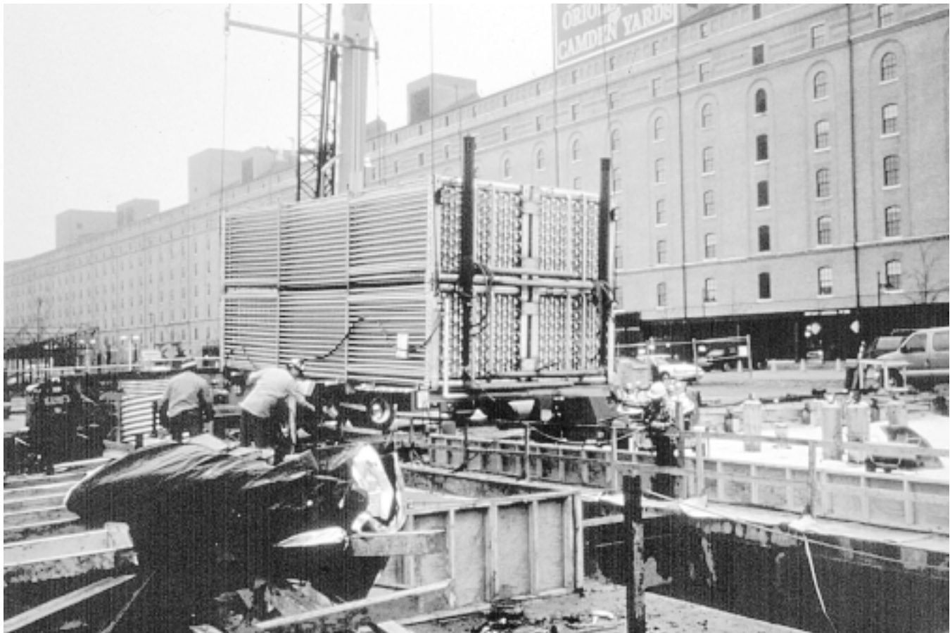
Fig. 10 An external-melt storage module for a district cooling system A large number of these modules are installed underneath a parking lot. The system serves a portion of downtown Baltimore.
