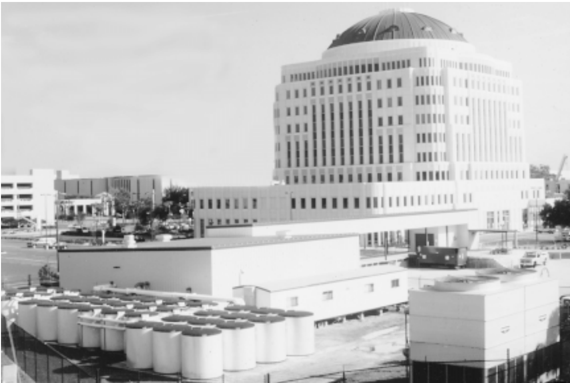
Fig. 14 A large modular coil-melt cooling storage system The storage units are installed on grade, outside the low mechanical equipment building. The system serves the large domed building in the rear.
