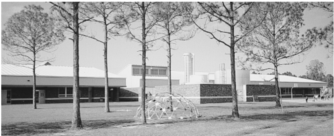
Fig. 16 Separated ice slurry cooling storage system The system provides air conditioning for an elementary school. The storage equipment is surrounded by the brick enclosure in the foreground.
