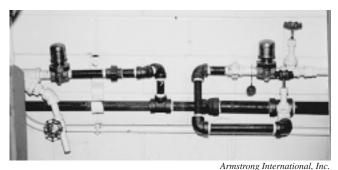
Fig. 7 A pair of thermostatic wafer steam traps The main attraction of these is their small size and low cost.
