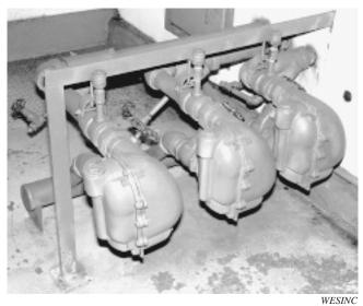
**Fig. 3 Typical F&T traps** The chubby shape provides space for the float ball to swing up and down. The thermostatic element is on the upper left.
