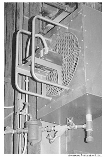
Fig. 5 A small inverted bucket trap draining a steam-fired space heater
