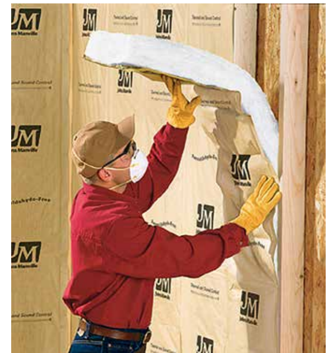
Figure 3-36. Glass fiber batt being installed in a frame wall. Note that the tabs of the backing sheets are overlapped properly, creating an unbroken vapor barrier.
