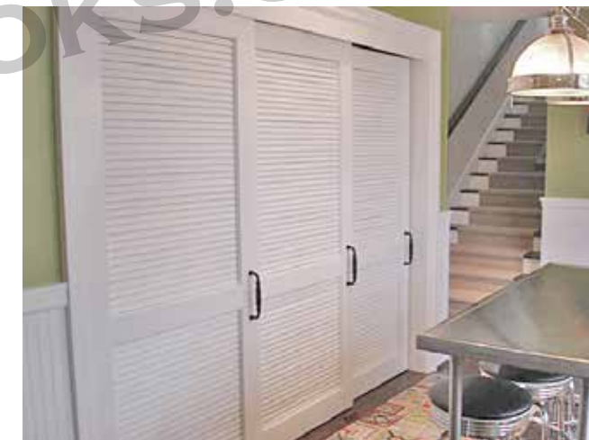
Figure 3-245. An attractive set of sliding doors for a closet.
