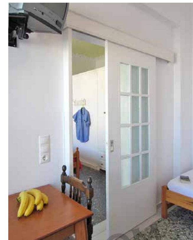
Figure 3-244. An interior sliding door with glazing.
