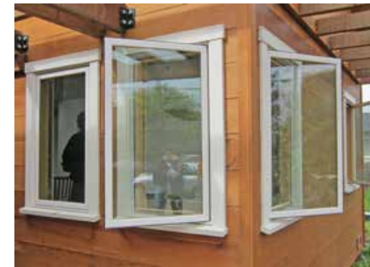
Figure 3-204. Casement (Outward Swinging)
