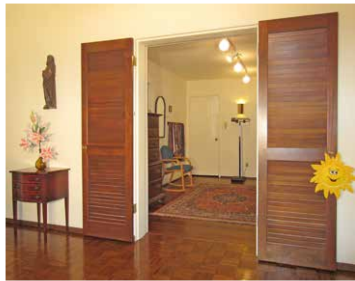
Figure 3-242. Louvered doors between a bedroom and a dressing room.
