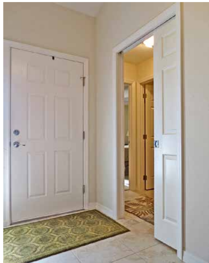
Figure 3-243. A pocket door that isolates a bedroom wing from the rest of the house. This style of door mounting avoids interference with the bedroom hallway and with the entrance door on the left.
