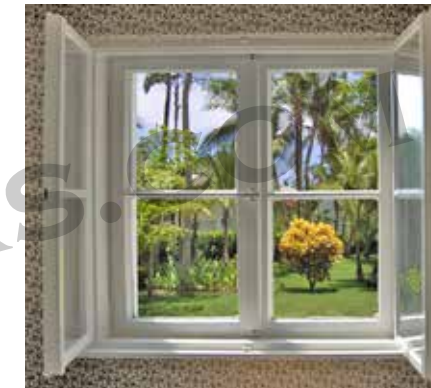
Figure 3-205. Casement (Inward Swinging)
