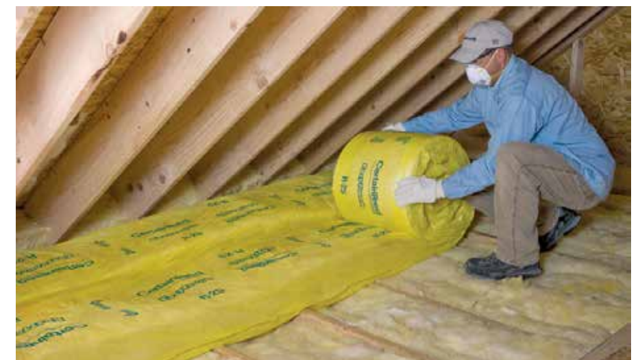
Figure 3-37. Proper installation of batt insulation in an attic. The upper layer or layers must have no vapor barrier, so that moisture can vent into the attic space. The crisscrossed arrangement of the batts provides optimum resistance to heat leakage along the joists and between the batts.
