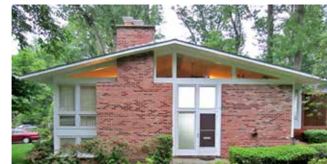
Figure 2-36. The clerestory windows in this gable end wall are well shaded by a deep roof overhang. The result is diffuse daylighting with little solar heat gain. This is efficient for a warm climate, but not for a cold climate.
