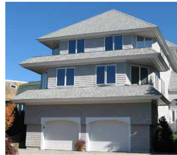
Figure 2-17. False eaves on a Florida house. At this sun angle, approximately half of the window area is shaded.
