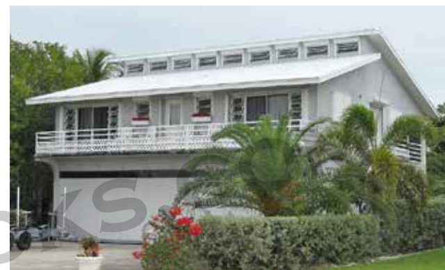
Figure 2-34. A house in the Florida Keys with clerestory windows that provide ventilation as well as daylighting. This arrangement provides daylighting for the rooms at the rear of the house.
