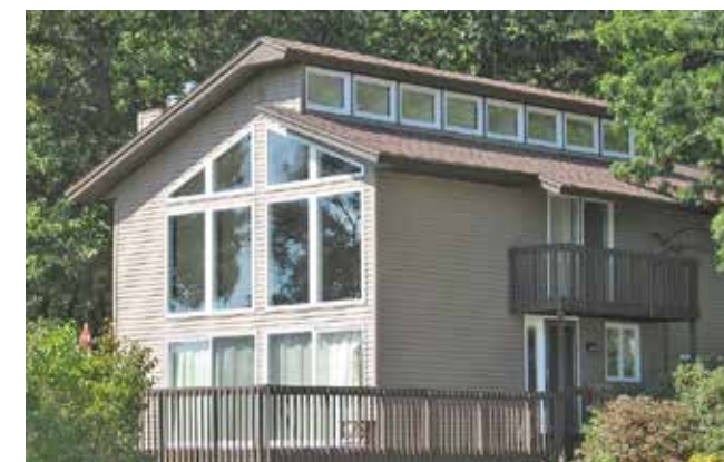
Figure 2-37. This house has two sets of clerestory windows. One is between the roof planes. A triangular clerestory is located over the main windows in the side wall.
