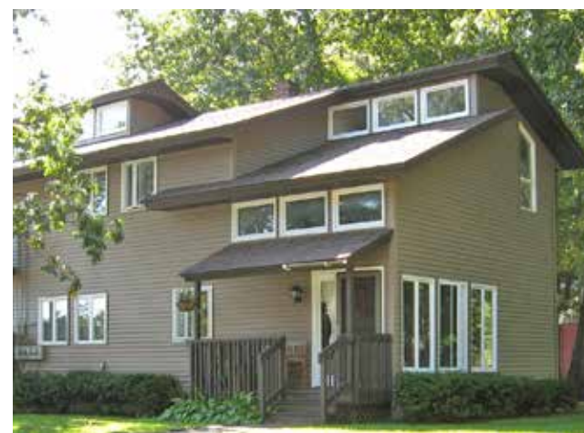
Figure 2-35. The upper clerestory, between the two roof planes, provides daylighting for the rear of the house. The clerestory over the front porch provides daylighting for the front of the house.
