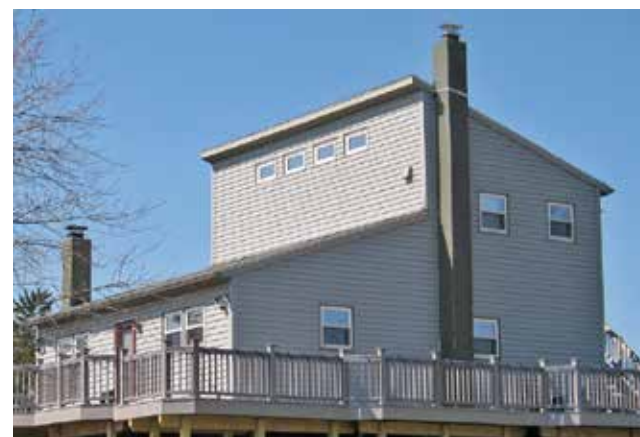
Figure 2-33. Clerestory windows along the top of the high wall under a shed roof. This style is effective for daylighting, but austere in appearance.
