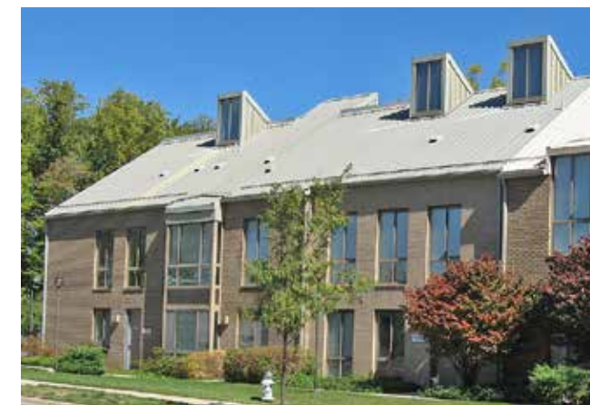
Figure 2-38. Clerestories created by extending the roof rafters beyond the ridge. These create a somewhat bugeyed appearance.
