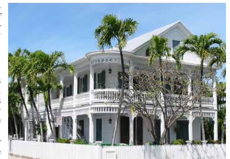
Figure 2-18. A house that uses both a porch and a balcony for effective shading.
