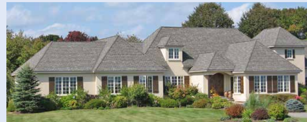
Figure 1-197. Hip roof. A gable roof that has hips, which are sloped ends, instead of gable end walls. Primarily an appearance feature. For good appearance, the hips generally have the same slope as the main gable. Can be built with truss or triangle-frame construction. Sacrifices valuable attic space. Complicates the carpentry somewhat. Considered to be less vulnerable to wind damage than a simple gable shape, although both styles resist wind damage if they are built strongly.
