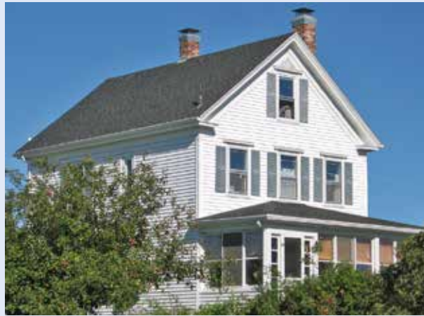
Figure 1-190. Gable roof. This is the basic shape for most roofs because it is strong and easy to build. Usually, the sides are symmetrical. The eaves can be extended easily to provide wide overhangs.
