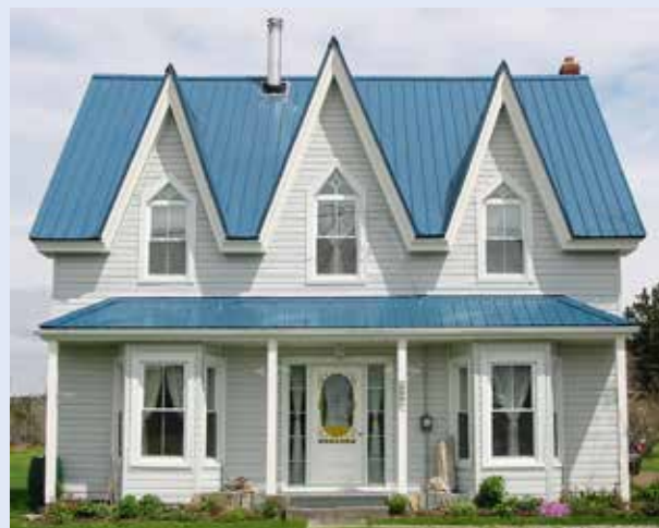
Figure 1-192. Side gables provide daylight, view, and additional living space, usually in roofs with triangle-frame construction. The side gables may have the same height as the main gable or they may be shorter. Shorter gables tend to weaken the portion of the roof where they are attached.
