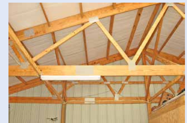
Figure 1-108. This truss roof uses purlins to support a sheetmetal surface, increasing the distance between the trusses.
