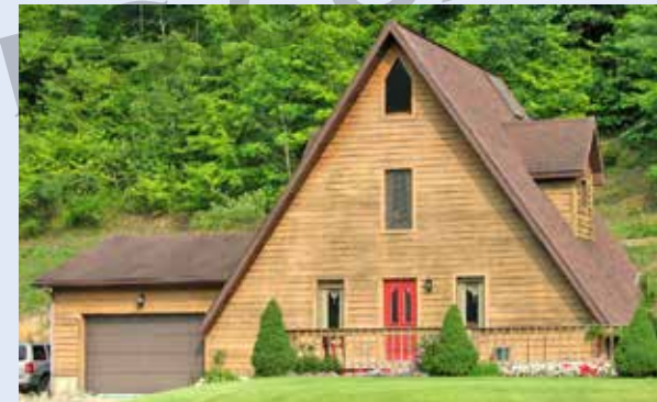
Figure 1-196. A-frame roof. This roof structure encloses the entire house. It may have one or more floors of living space. The rafters function as wall studs, usually resting on a short foundation. Dormers may be added to provide daylighting and view through the roof surfaces.
