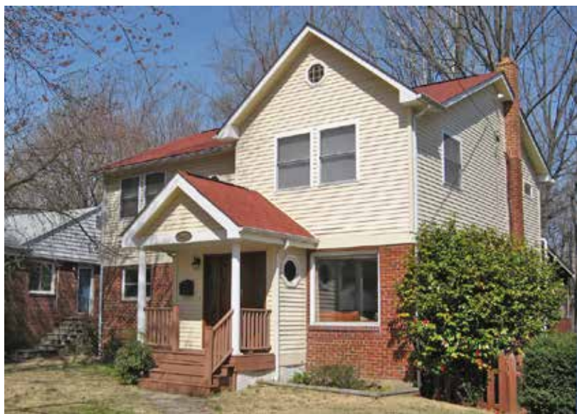
Figure 1-124. An attractive second story addition. The result matches the original style well. The house was originally identical to the one at its left.
