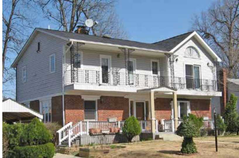
Figure 1-125. Another attractive second story addition.
