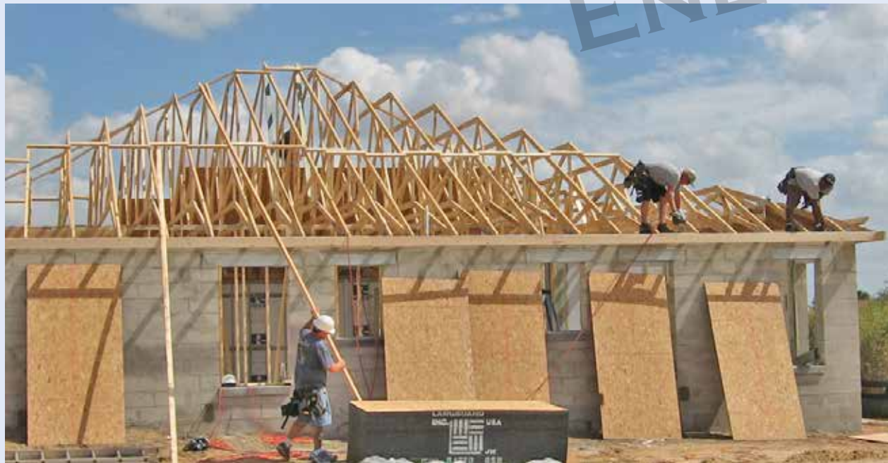
Figure 1-106. A truss roof being built. It is about to be covered with the sheathing panels that are stacked along the wall. Note the variety of truss shapes needed to create a “hip roof” shape.
