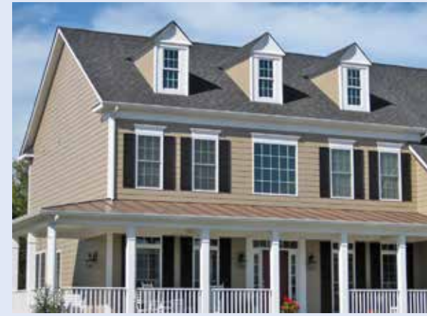
Figure 1-194. Dormers provide increased daylight and view through the sides of a triangle-frame roof. They can serve as clerestories for a beam roof. The width of dormers is limited, to avoid weakening the roof. Dormers can be effective appearance enhancements to break up a large roof surface.
